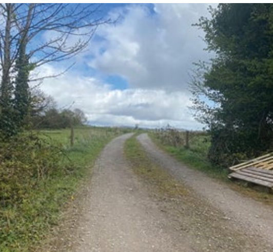
A builder built an extra thirteen houses in an existing housing estate. The builder rerouted heavy traffic away from the estate and used an existing farm road at the rear of the site to access the building site. The photo shows the relief road and this road was in existence long before his company built these houses. After the houses were built the Council instructed the builder to go onto private property and dig up the relief road and turn the area into a green field otherwise Kerry County Council will take €20,000 via a bond from the builder. Kerry County Council contacted this publication stating that the heading of this article is "grossly misleading and incorrect". Nobody wants badly built estates but this example does not entice builders to build houses.
