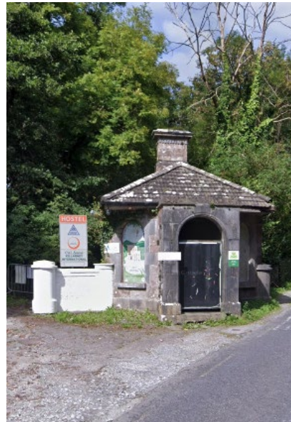
Gate Lodge at Aghadoe House, Knoppogue, Aghadoe, Killarney will receive €13,360.97
