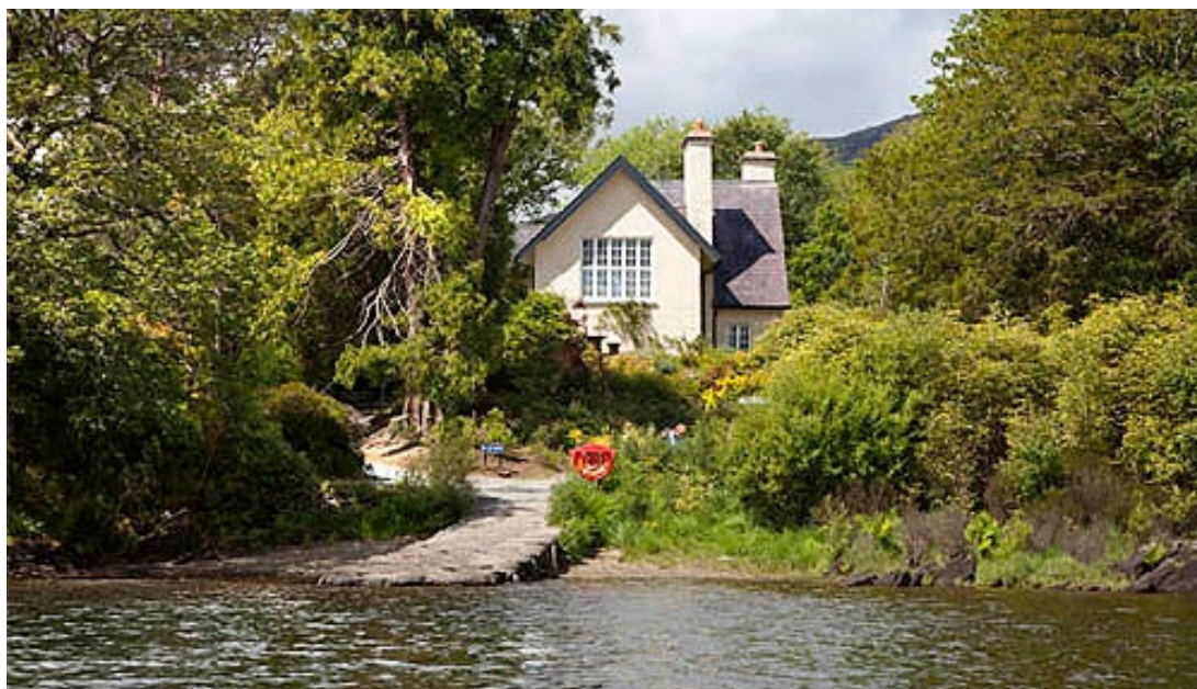
Following the granting of planning permission Dinis Cottage will now be accessible for walkers and cyclists by a raised platform from Torc.
